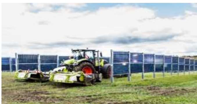
Fig 2. Vertical solar panel
