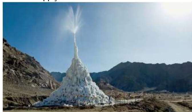
Fig 2: An Ice Stupa in Ladakh accumulates ice from a sprinkler-like system (K Lyons, 2023)
